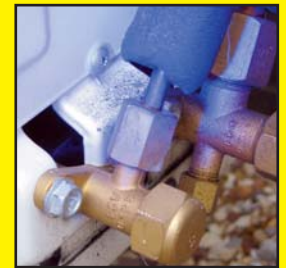
The site is then re-inspected with the lamp. No glow means that all leaks were repaired successfully
